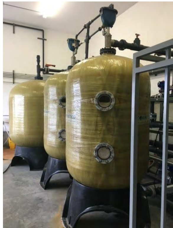
Arsenic Treatment Plant
