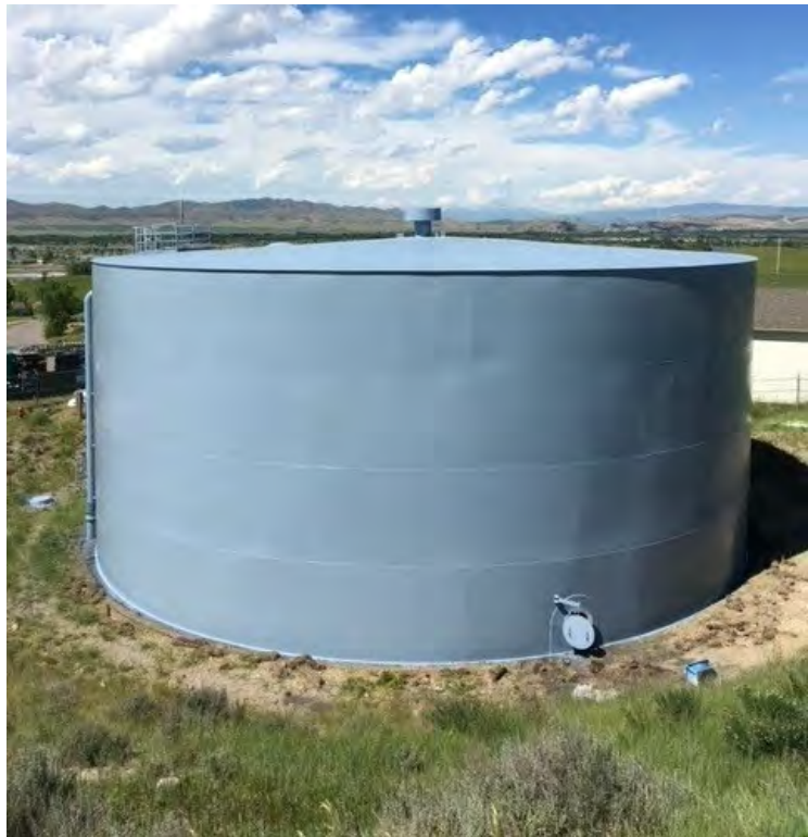
1-Million Gallon Welded Steel Water Storage Tank
