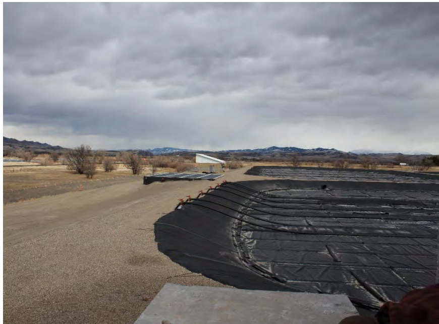
Treatment Lagoons, Polishing Reactor, and UV/Blower Building
